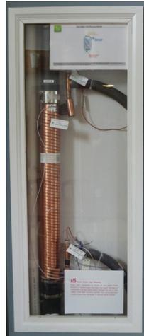
Figure 1. Drain water heat recovery unit at Archetype House B
