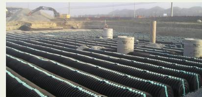
*Infiltration chambers can be designed for full infiltration, partial infiltration or partial infiltration with flow restrictor. Exploring these options for designs on low-permeability soils would provide stormwater runoff benefits to otherwise underutilized locations.*
