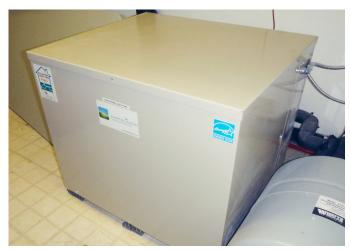
Figure 1. DX ground-source heat pump in basement mechanical room of House A.
