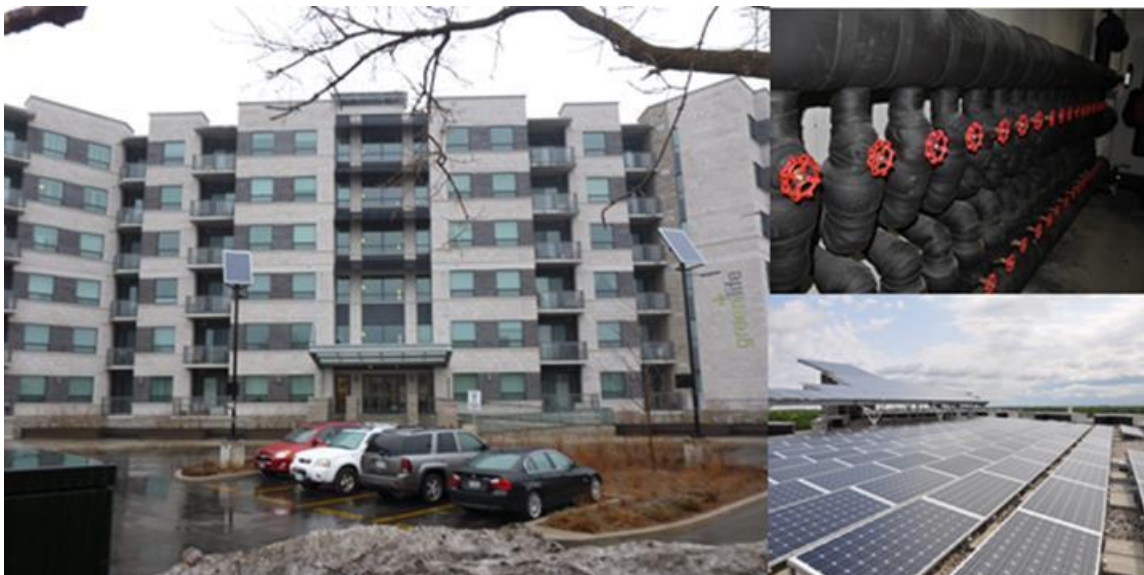
Figure 4.17: (Left) Front view of the Greenlife condominium. (Top right) Part of the ground loop manifold located in the basement parking garage. (Bottom right) Part of the solar photovoltaic system on Greenlife's roof.
