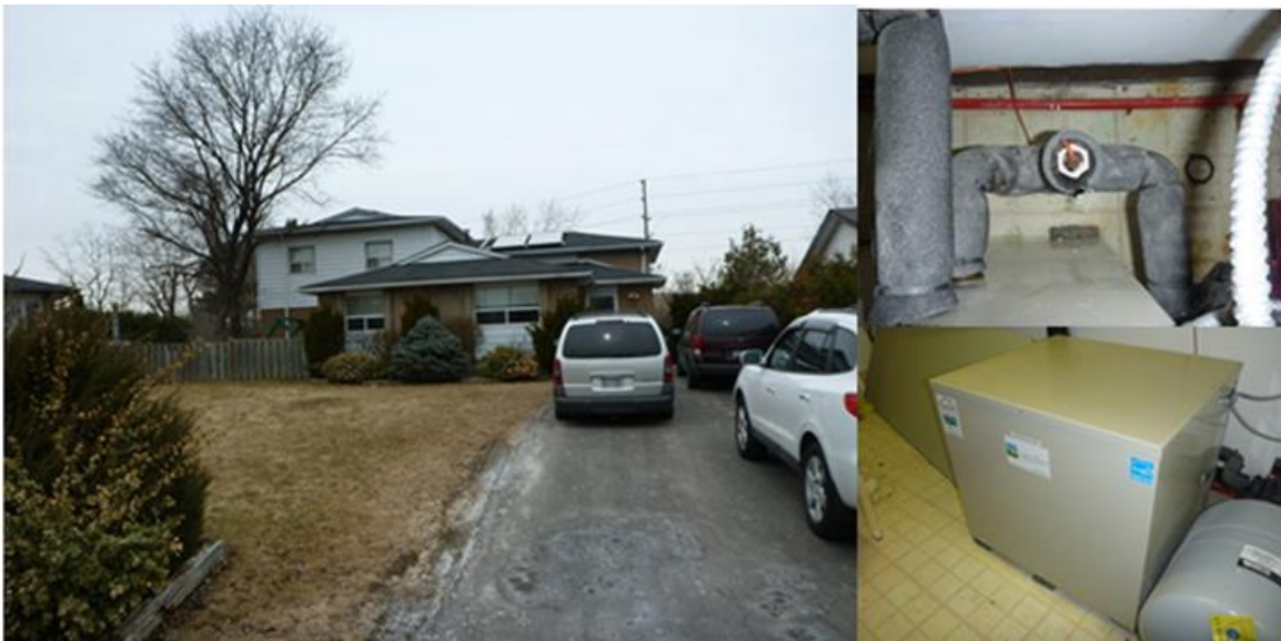
Figure 4.1: (Left) Street view of Peel House A. (Top right) A resistance temperature detector (RTD), used for temperature monitoring, installed in a thermal well. (Bottom right) The heat pump compressor box.
