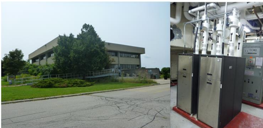
Figure 4.34: (Left) Street view of the Downsview Park Office Building. (Right) Two TMW 340 Climate Master heat pumps power the georexchange system.
