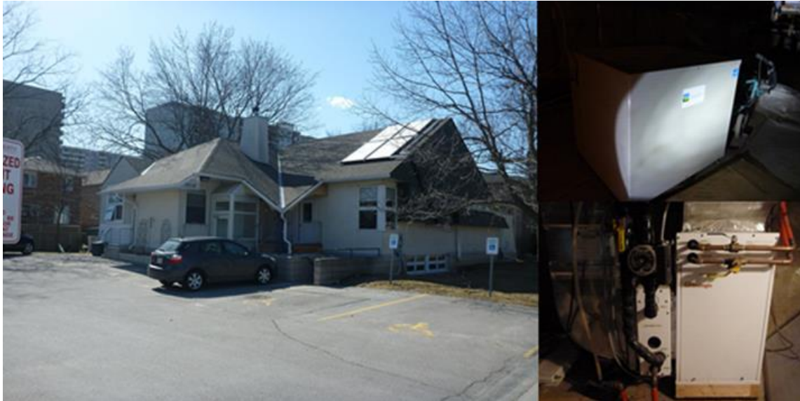
Figure 4.9: (Left) Street view of Peel House B. (Top right) Compressor box of ground source heat pump. (Bottom right) Air handler with hydronic coil.
