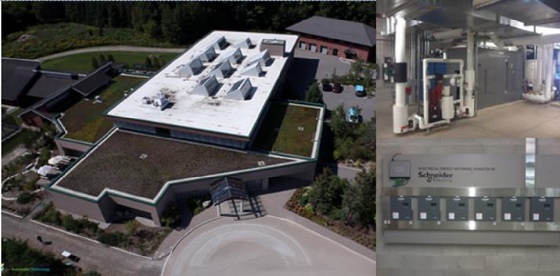
Figure 4.49: (Left) Aerial view of Earth Rangers Centre showcasing reflective white roof, green roof and solar thermal panels. (Top right) Ground source heat pump in mechanical room. (Bottom right) Energy monitoring boxes.
