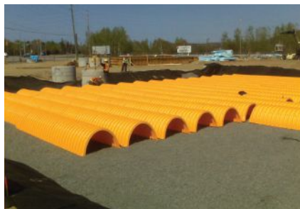
Underground infiltration systems can be effective on fine-textured soils at maintaining pre-development groundwater recharge with thoughtful design.
