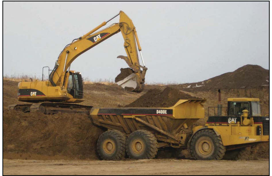
How topsoil is stripped and stockpiled affects its composition, structure and moisture holding capacity.
