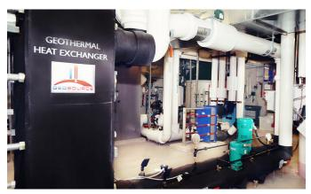
Figure 1. The geothermal heat exchanger in the basement mechanical room of the Earth Rangers Centre for Sustainable Technology.
