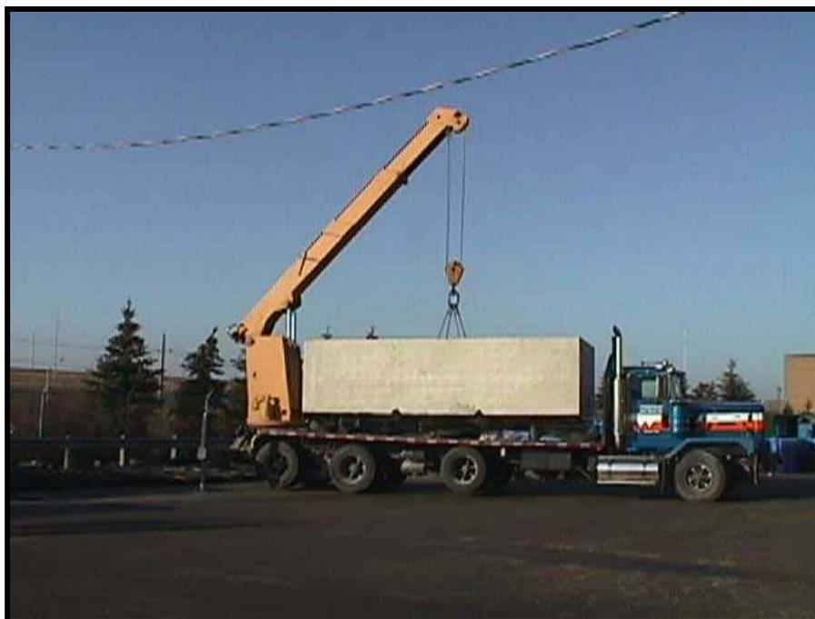
**Figure 4.10:** Installation of the Off-line Sediment Holding Tanks
