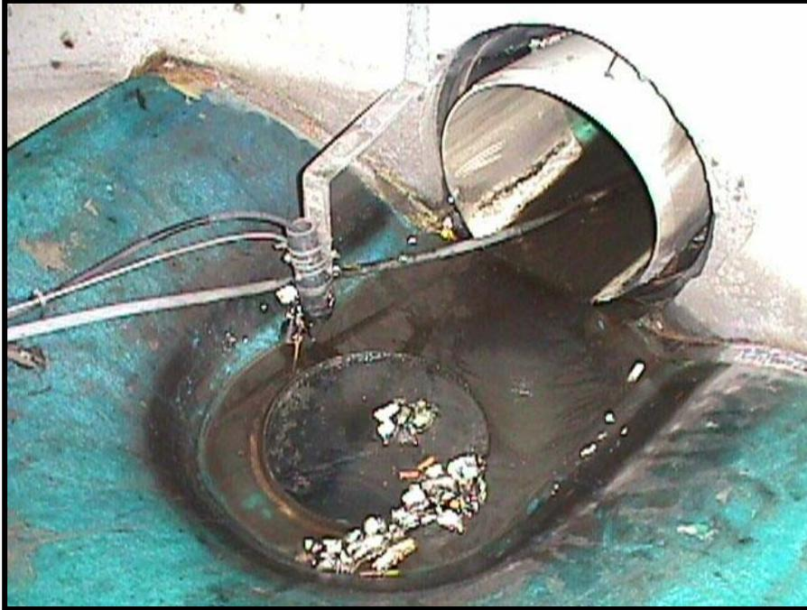
**Figure 4.6:** Monitoring Equipment Installed at the Stormceptor Weir
