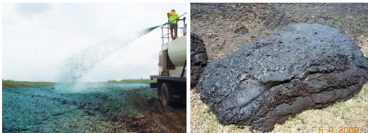
Figure 1.5: Application of hydroseed mixture with PAM (left) and thickening effect of PAM on wet sediment (right, courtesy Applied Polymer Systems Inc.)
