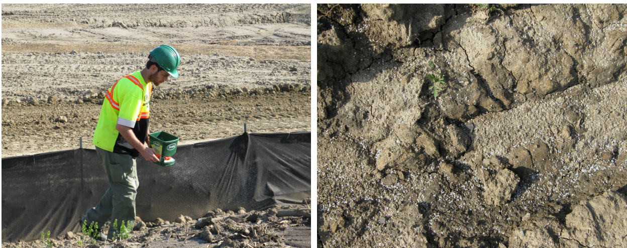
Figure 2.1: Application of granular anionic PAM to a construction site soil stockpile
