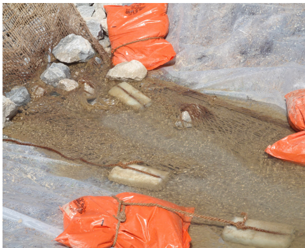
Figure 2.2: TRCA evaluation of anionic PAM for water clarification in a ditch
