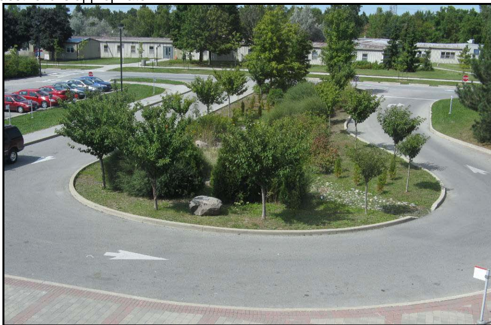
Figure 10 – Bioretention cell at York University, Toronto, ON (Source: TRCA)
