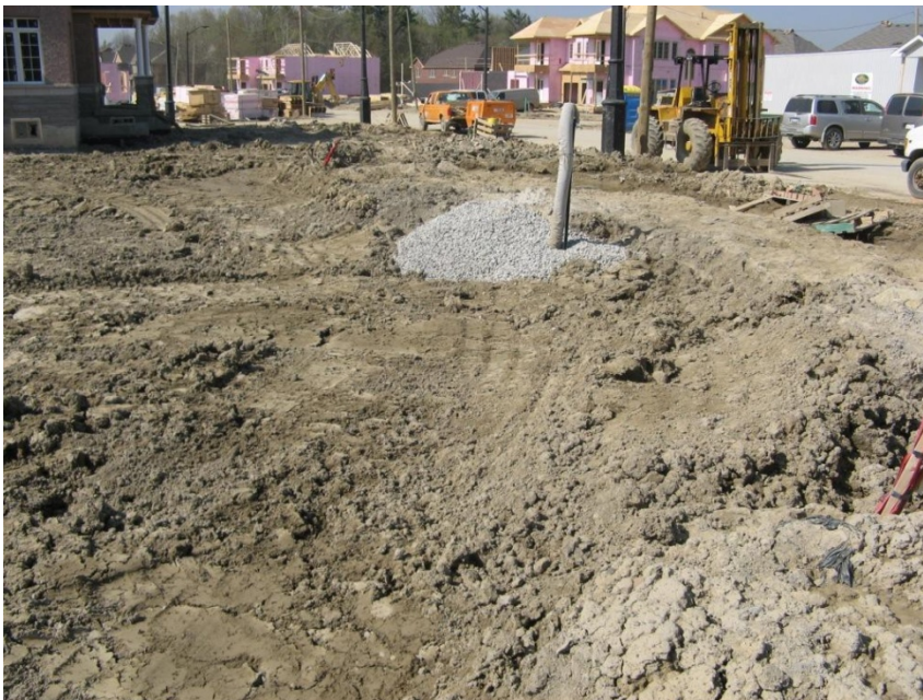
Figure 2.7: Stormwater ponding area at the study site during home construction
