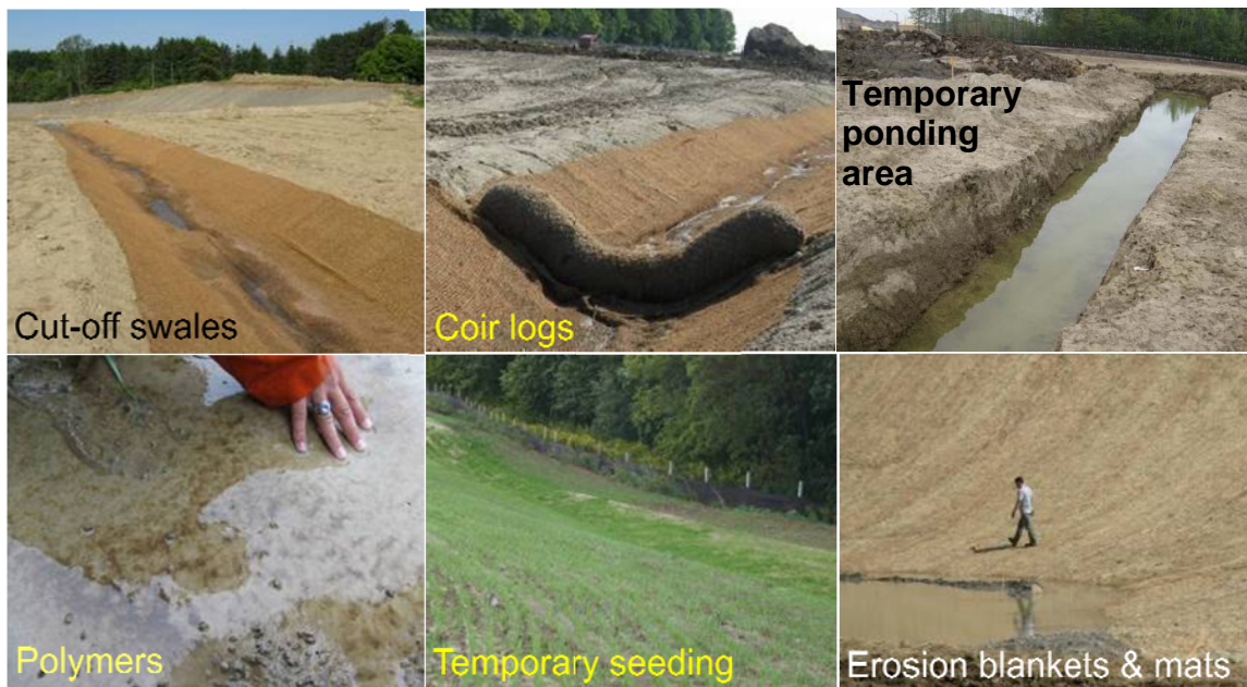
Figure 2.2: Examples of ESC Measures installed at the Block 39 study site
