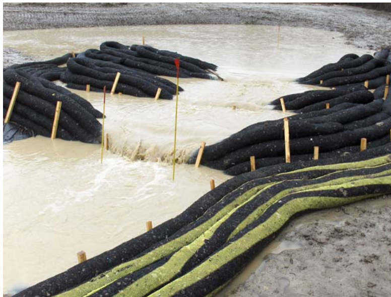
Figure 38: Biofilter overflow caused by high flow rates, December 1, 2006 13:05 pm.
