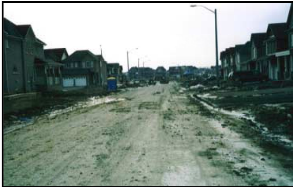
Figure 5: Road conditions in Catchment-1070 during construction
