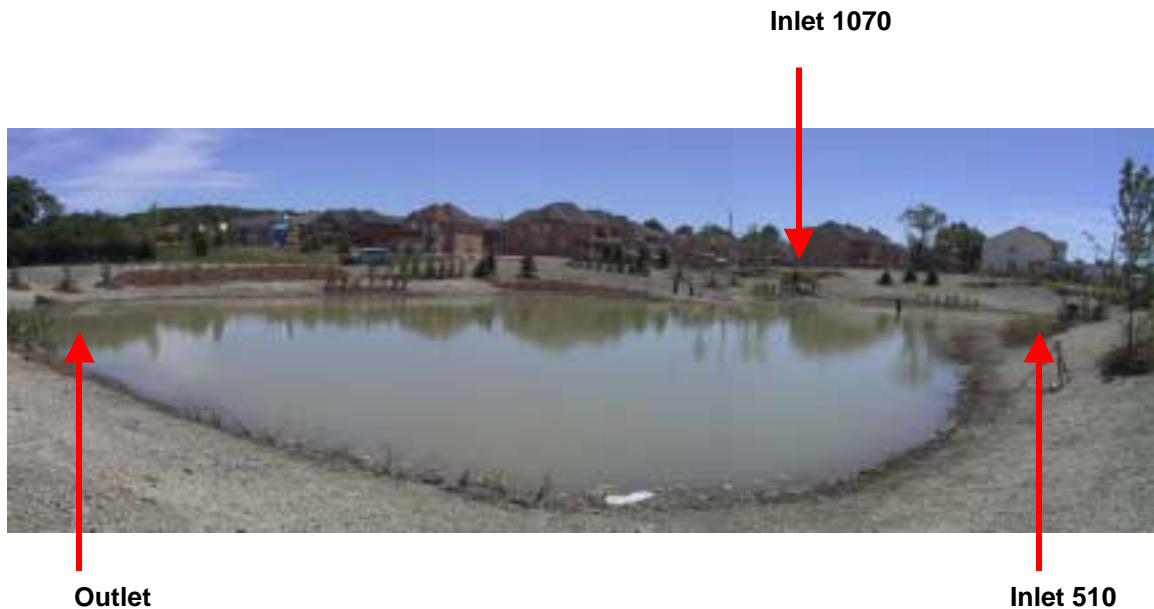
Figure 2: Ballymore sediment control pond
