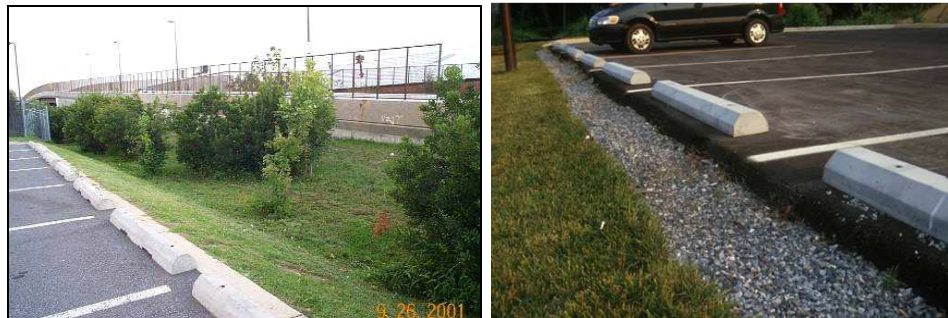
Figure 4.6.3 Filter strips providing pretreatment of parking lot runoff
