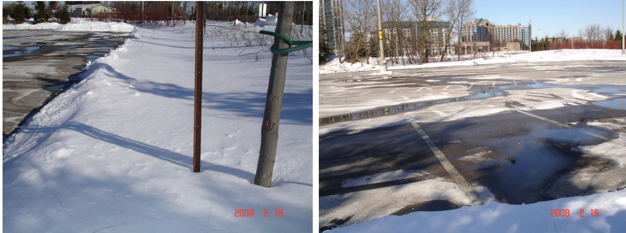
Figure 4.6.2 Snow storage on a filter strip in Markham, Ontario
