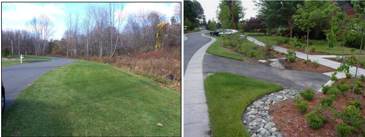
Figure 4.6.1 Filter strips along a residential road and as pretreatment to a dry swale
