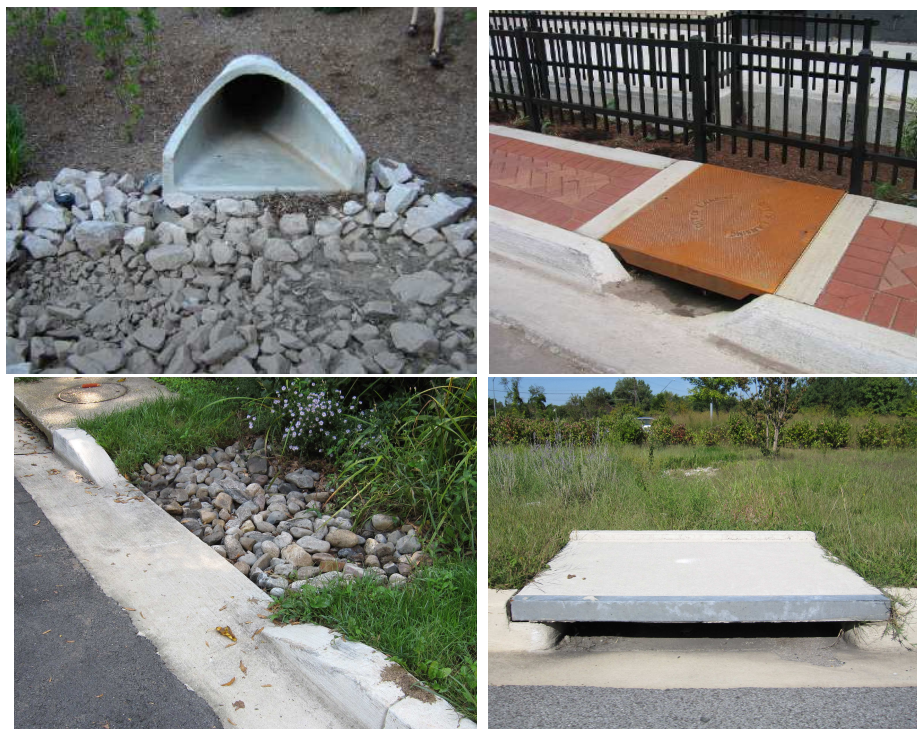
Figure 4.5.10 Examples of inlets to bioretention practices
