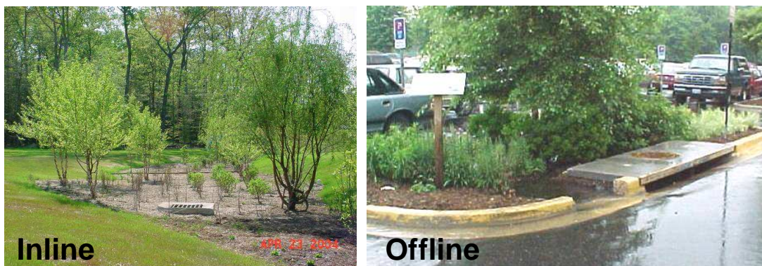
Figure 4.5.9 Examples of inline and offline bioretention
