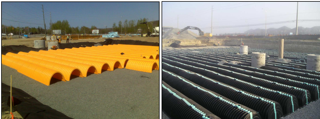
Figure 4.4.2 Infiltration chambers under construction in commercial developments
