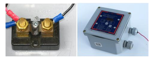
**Figure 3.1:** Amp meter shunt used to measure electrical current to and from the batteries (left). Battery meter logs data collected by an amp meter shunt (right)
