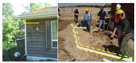
Figure 1-1. [LEFT] 1. Gutter and 2.Downspout; [RIGHT] Conveyance drainage piping for below-ground rainwater storage tank (prior to burial)
