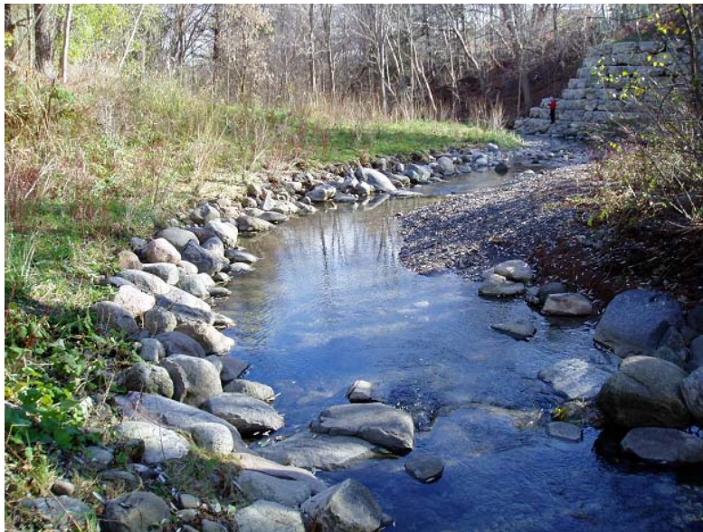
View of channel looking downstream. Note: well developed point bar and minor erosion behind rock treatment. Vortex weir (foreground) appears to be functioning as intended.
