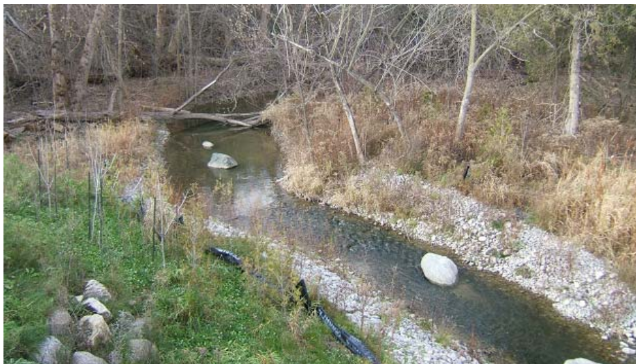
View of channel looking upstream. Note: vegetated rip rap lining both banks.
