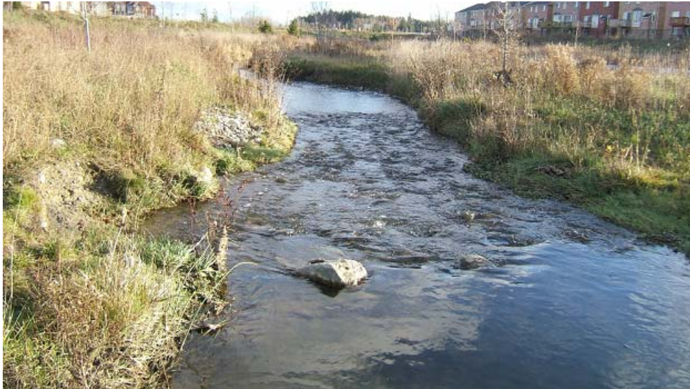
View of channel looking downstream. Note: riffle section appears to be functioning as intended. Some bank erosion and outflanking seen along left bank.
