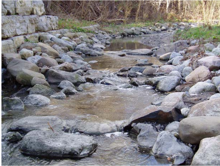
View of channel looking upstream. Note: well developed pool riffle sequences. Vortex weirs appear to be functioning as intended.
