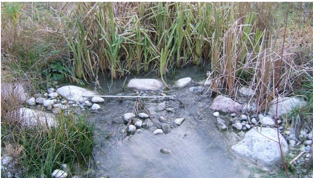
Partially exposed vortex weir and riffle viewed upstream. Note the in-channel vegetation in the upstream pool.
