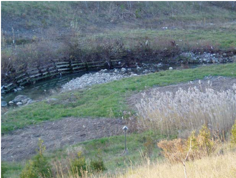
One of several cribwalls installed between Bellamy Road and Markham Road.
