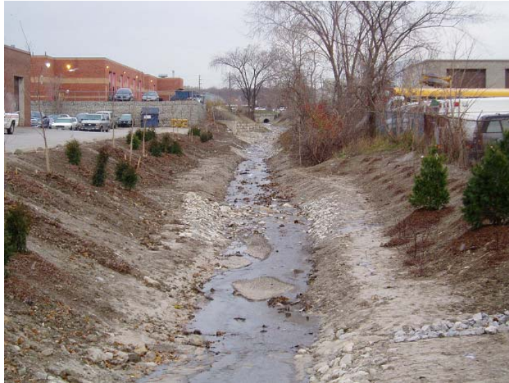
View of channel looking upstream. Note: some channel adjustments occurring since construction (medial bars and sediment deposition).
