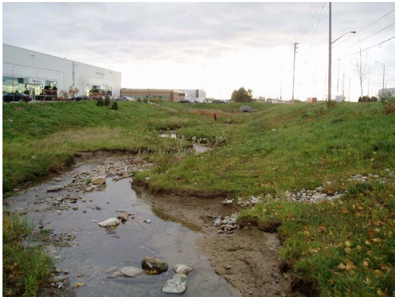
View of channel looking downstream. Note: extensive bank erosion and downcutting.
