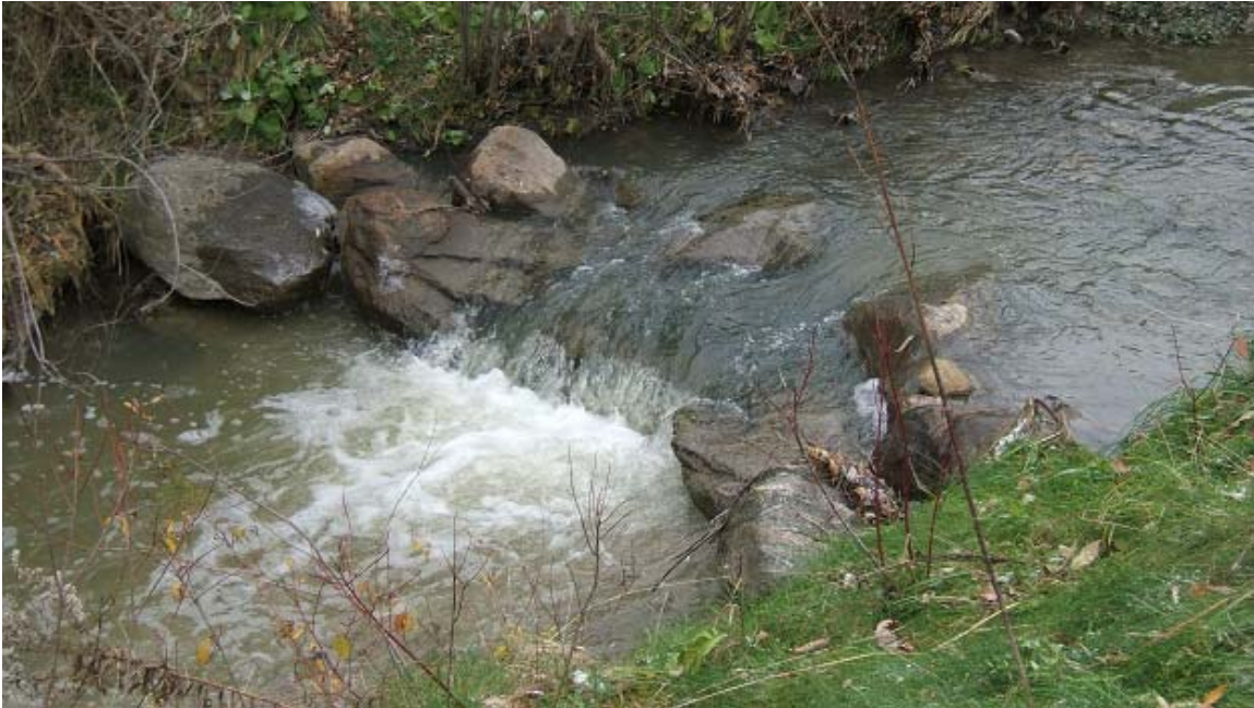
One of ten rock vortex weirs used for grade control.
