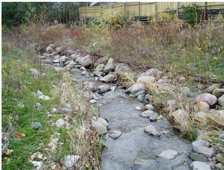
View of channel looking downstream. Note: fascines doing well along right bank.
