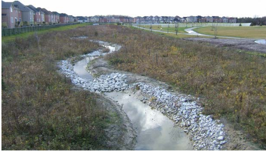
View of channel looking downstream. Note: riparian vegetation becoming well-established, rip rap placement and exposed riffle materials.
