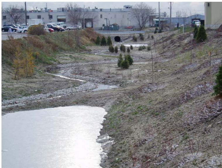
View of channel looking downstream. Note: newly constructed channel with low gradient and high sinuosity.
