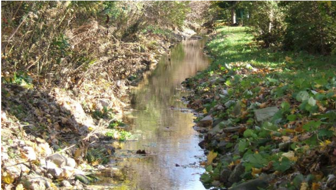
View of channel looking downstream. Note: vegetated rip rap (left bank) and rip rap and residential lawn (right bank).
