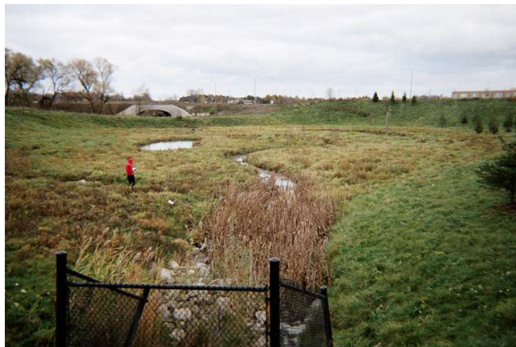
View looking upstream from most downstream extent of NCD. Note: wide floodplain, offline pond features, sinuous channel.
