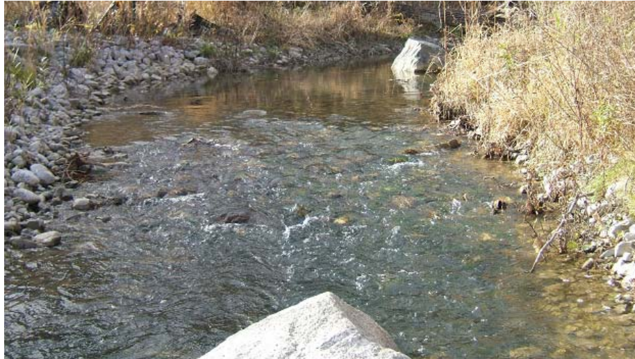
View of channel looking upstream. Note: riffle structure and boulder placement generally functioning as intended.
