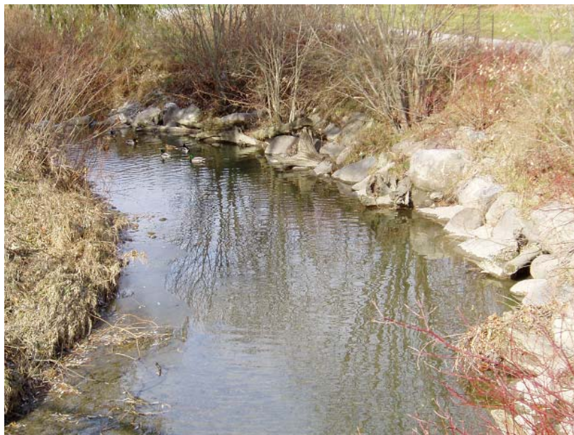
View of channel looking upstream. Note: vegetated rip rap (right bank) and root wad placement.
