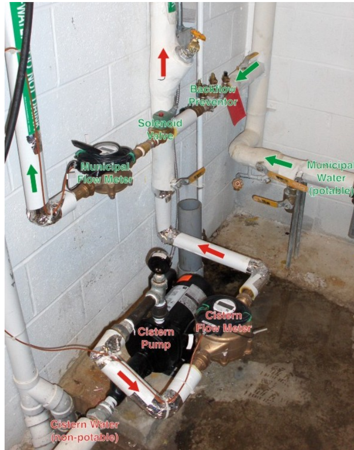
Figure 4.2: Flow meter schematic inside Metro Label printing facility.
