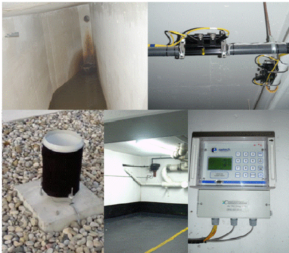
Figure 4.4: High rise apartment building monitoring equipment. Clockwise starting upper left—view inside the cistern; flow meters; logger; pump (black) for water from cistern; heated rain gauge.
