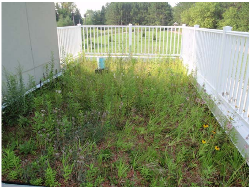
Figure 3.10: Green roof above House A garage
