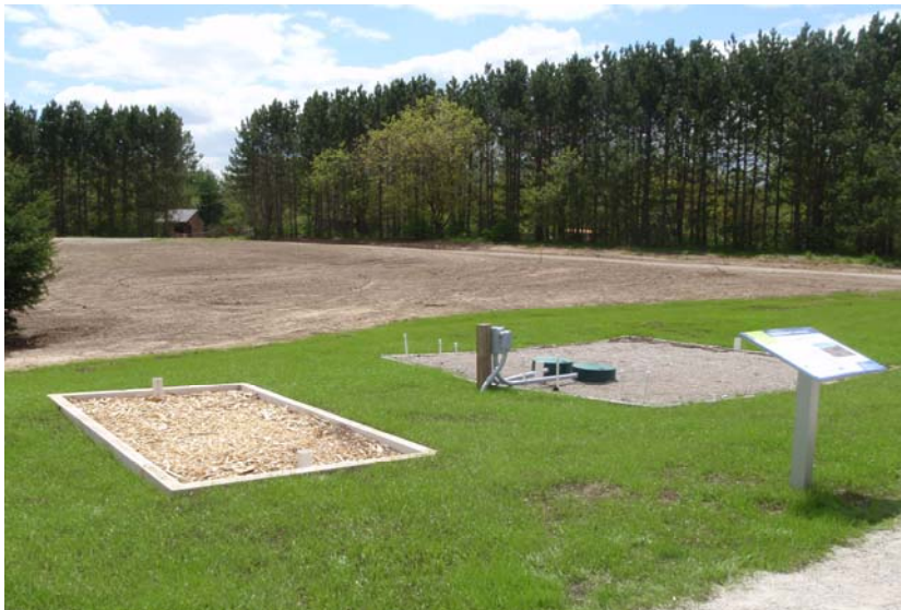
Figure 3.12: Surface view of the wetland wastewater treatment cells
