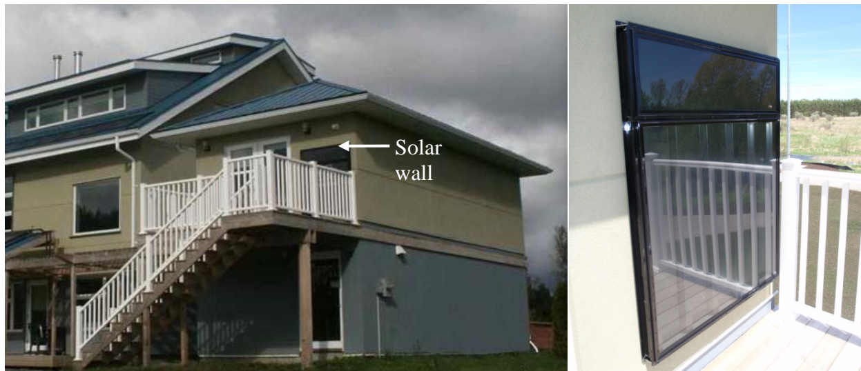
Figure 3.9: Guest suite of House B (left) and close up of guest suite solar wall (right)
