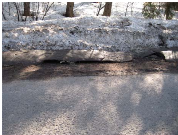
Figure 18: Dry road surface as surface water is retained by swale (MacFarlane, April 10, 2008)
