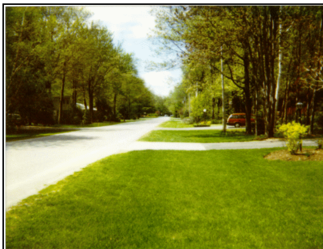
Figure 1: Streetscape of a typical grass swale and perforated pipe drainage system
