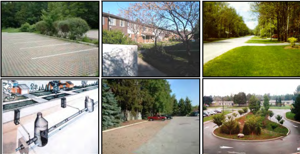
From top left to bottom right: Permeable Pavement at Belfountain Conservation Area (21 years), Green Roof over Below-ground Parking Garage at Gananoque Road Condominiums (30 years), Grass Swale and Perforated Pipe Drainage System in Ottawa (20 years), Exfiltration System in Etobicoke (17 years), Permeable Pavement at Jerrett's Funeral Home (14 years), Bioretention at York University (10 years).
