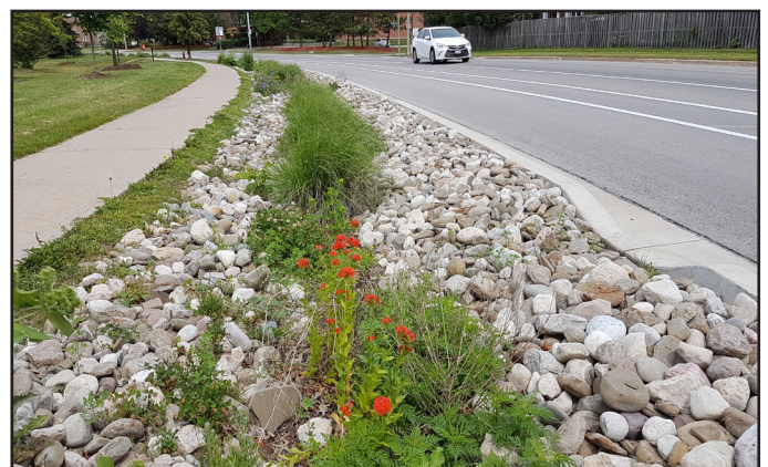
Figure 3. Biofilter swale retrofit within the road right-of-way
