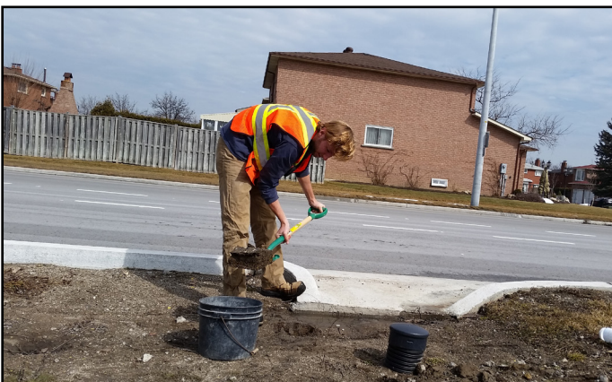
Figure 5. Sediment removal in Spring
